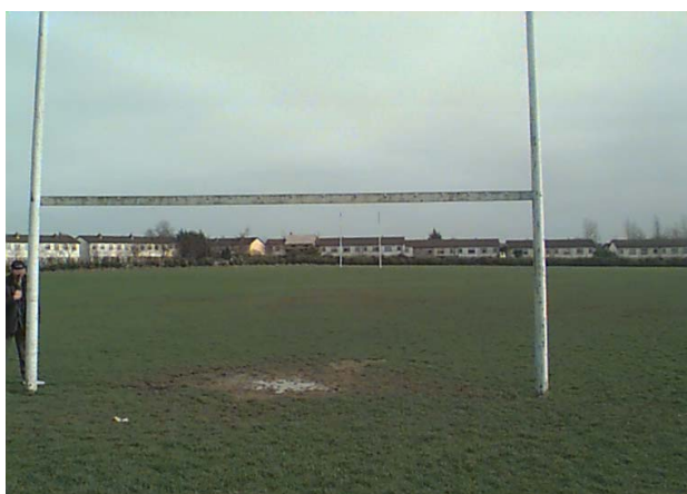
GAA goal post constructed of timber. Inappropriate for outdoor environments.
